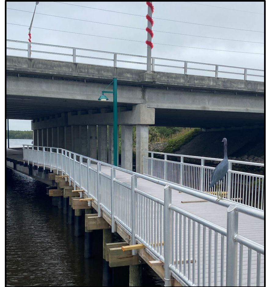
Eastern section of the bridge looking north (pre-construction)
