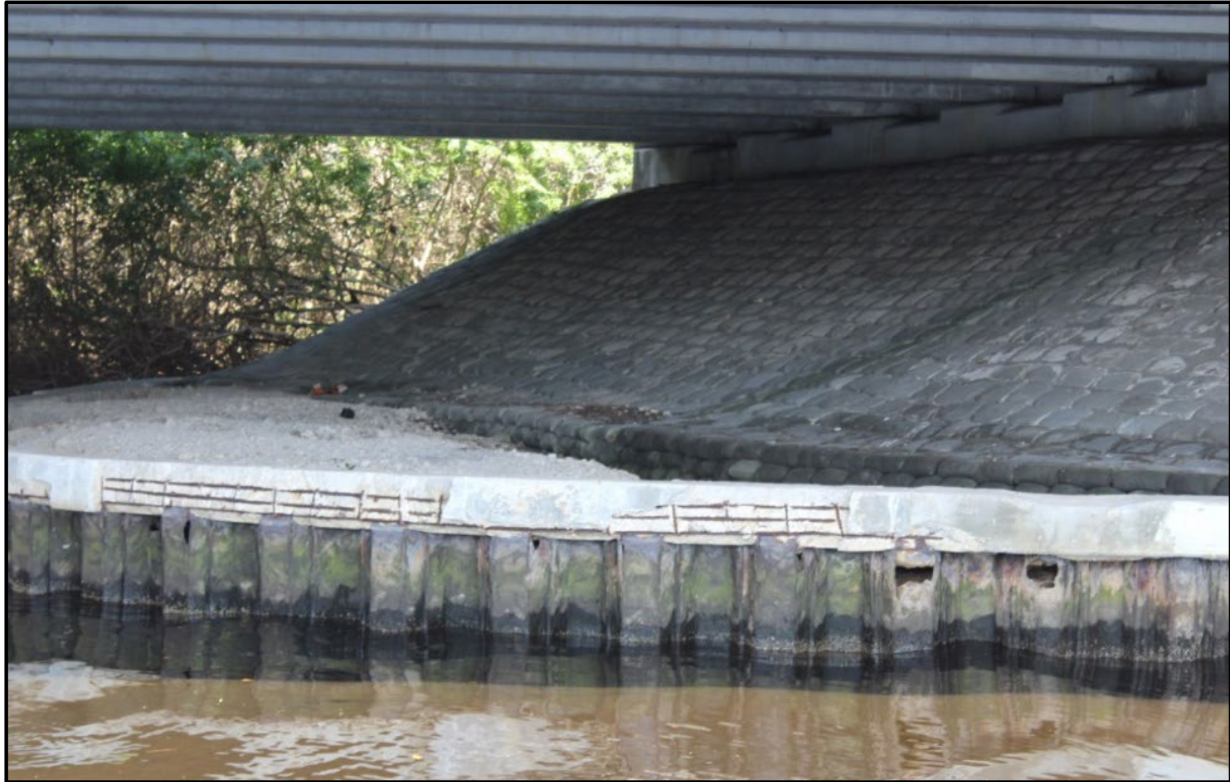
Existing view under the bridge (pre-construction)
