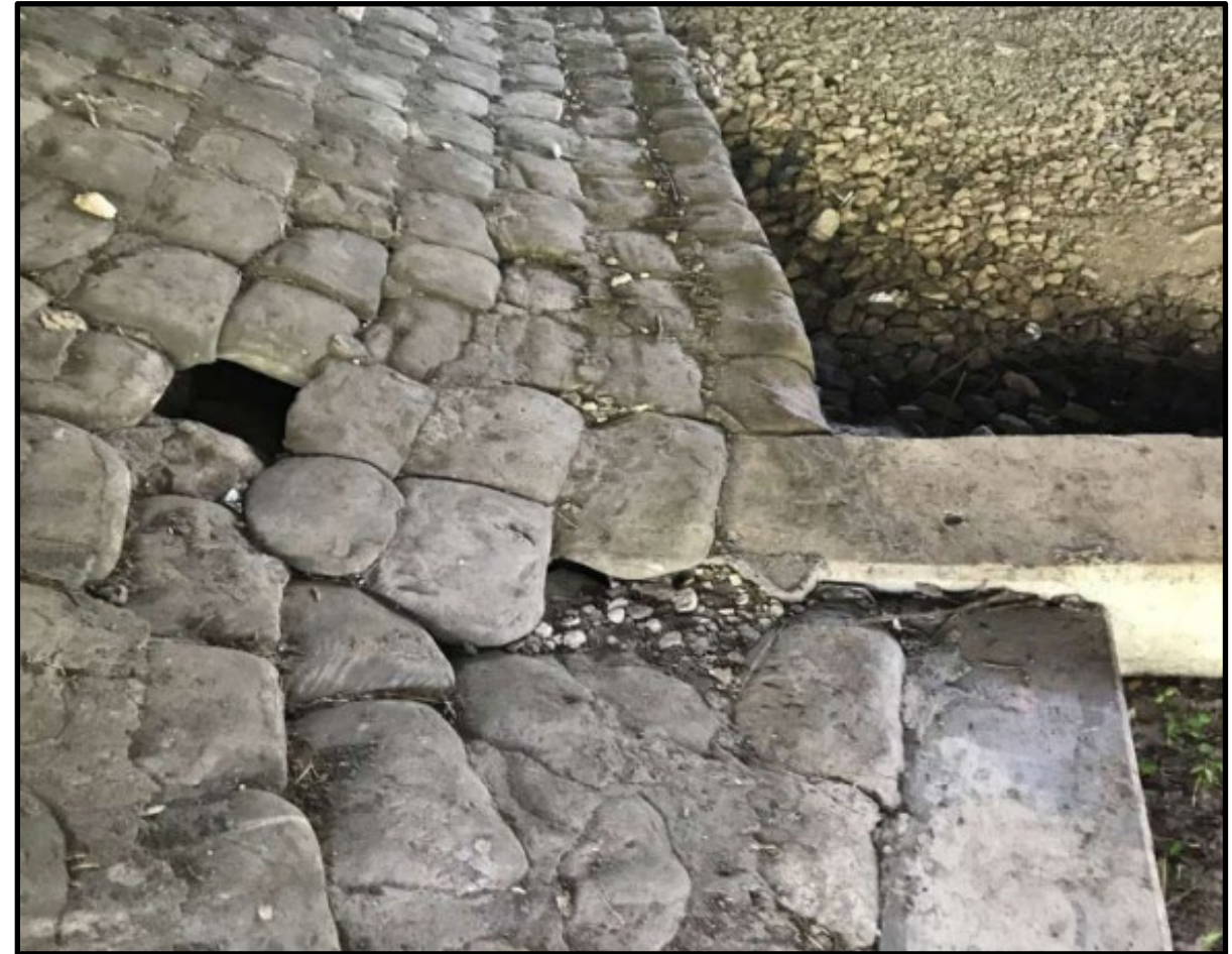
Existing sand-cement bags under the bridges (pre-construction)
